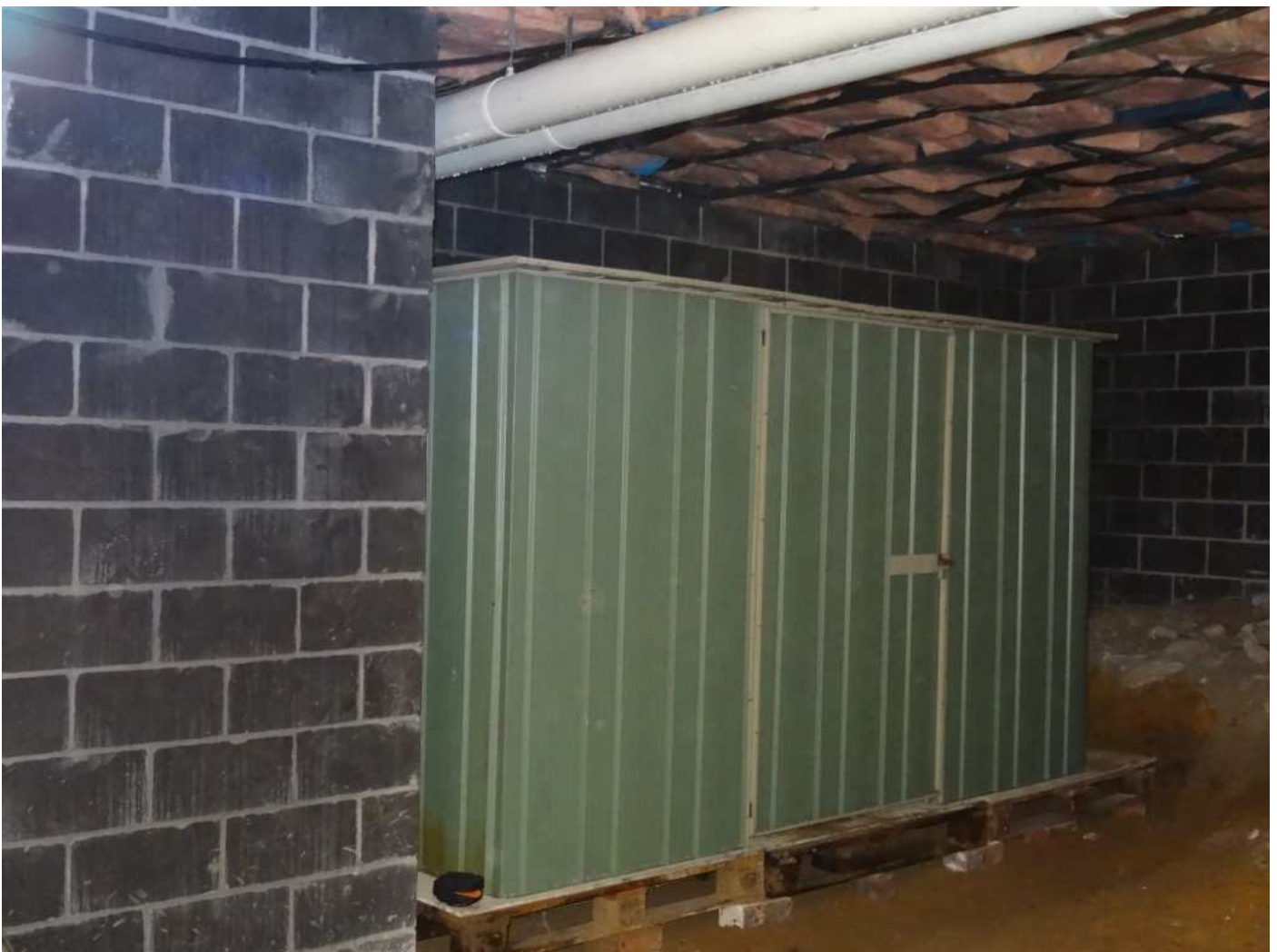
2014 – Club lockup shed donated by Milton installed in Church hall basement:
